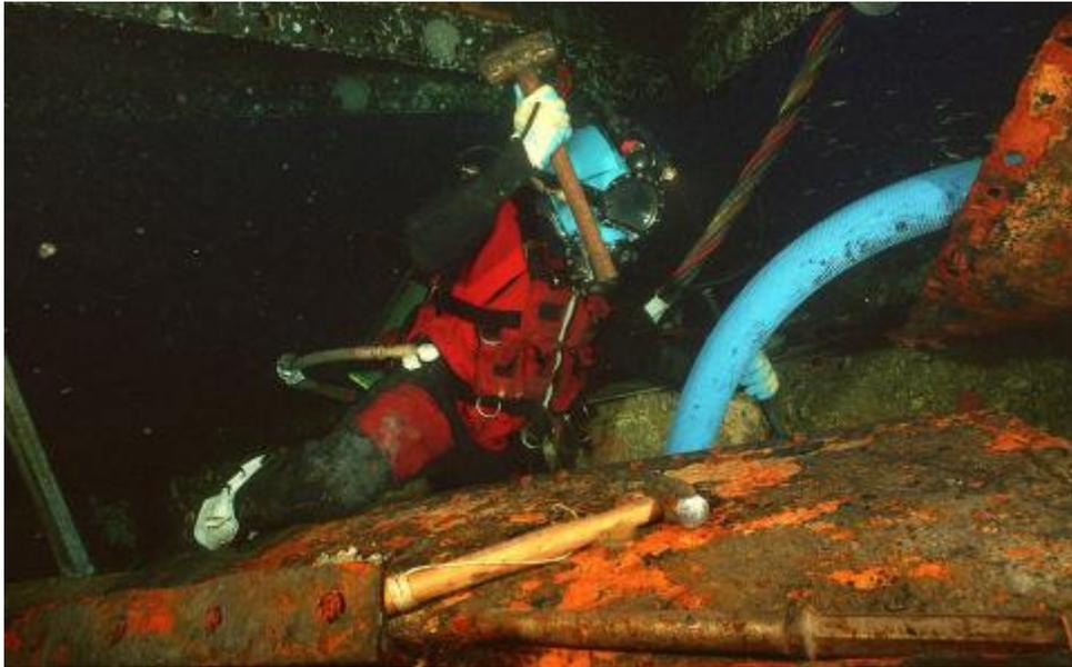
This U.S. Navy diver chiseling free deck plating from the sunken USS Monitor is an example of saturation diving, 2001.
